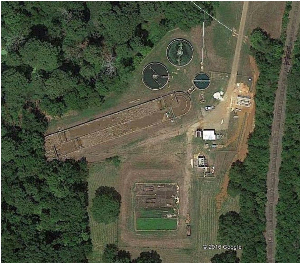
Figure 3.1 – Aerial Image of City of San Augustine WWTP
