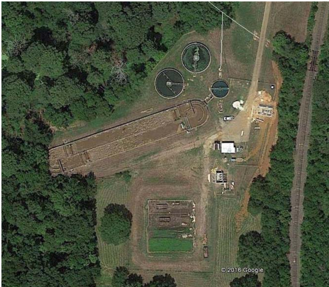
Figure 3-2: Aerial Image of the City San Augustine WWTP (Google Earth Image, 2016)
