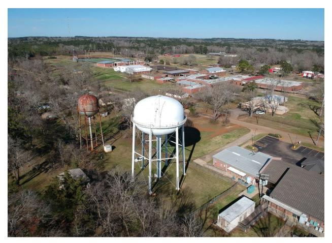
Caption: The water tower at the Hospital hold 500,000 gallons, and it floats on top of the distribution, meaning it only fills up when the pipes in the east side fill up first. It was a piece of equipment at the base that failed in the Ice Storm that caused so many of our problems.
