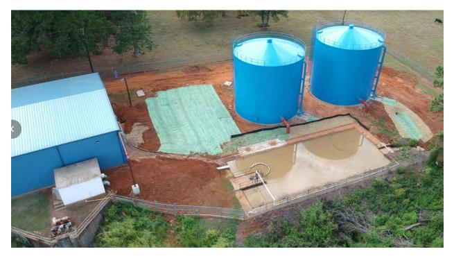
Caption: The 2 new 300,000 gallon water storage tanks (600,000 gallon total) were completed in 2019 to replace an old 500,000 gallon tank that was razed on completion after the new tanks went into service. The old tank could not be taken down for maintenance, but the new ones operate independently, so one can be worked on while the other remains working. The project was a major upgrade to the system.
