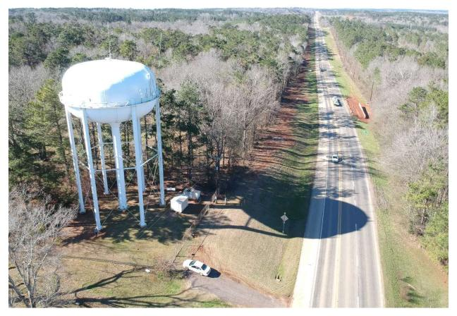
Caption: The water tower on Highway 96 also stores 500,000 gallons, and just like at the Hospital, it floats on top of the distribution, meaning it only fills up when the pipes in the west side fill up first. It is difficult to fill this up in normal times with the limitations of the City's pumping facility in mid-town.
