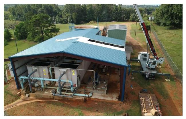
Caption: City Water Plant during a pump upgrade in August of 2019. If you count the grey pipes you can see they attach to basins 1 and 2. The plant was formerly outside, but has been enclosed in a building over the past few years. The building north end will be completed starting this spring.
