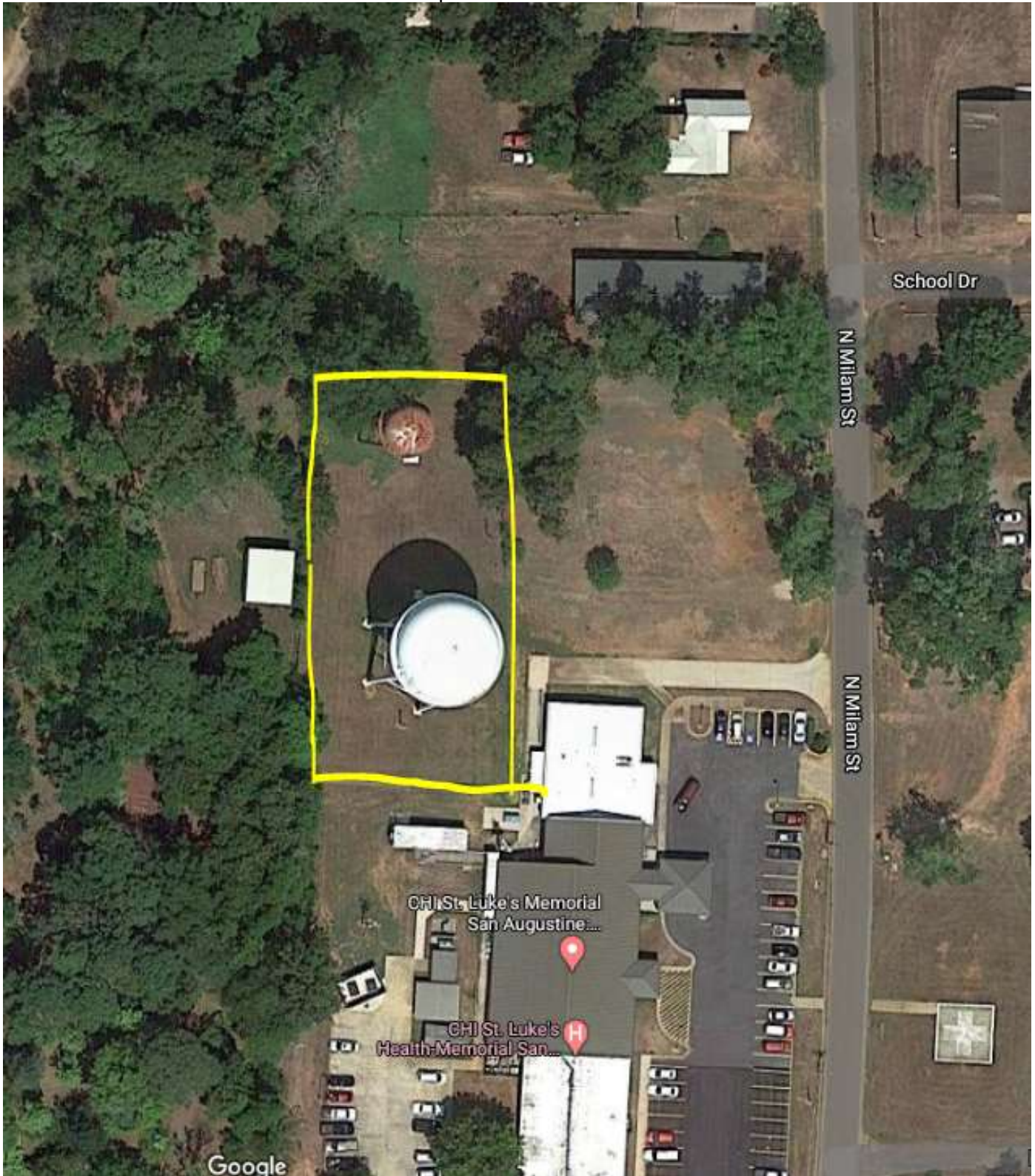
12. Water Tower on Milam St. behind the hospital
