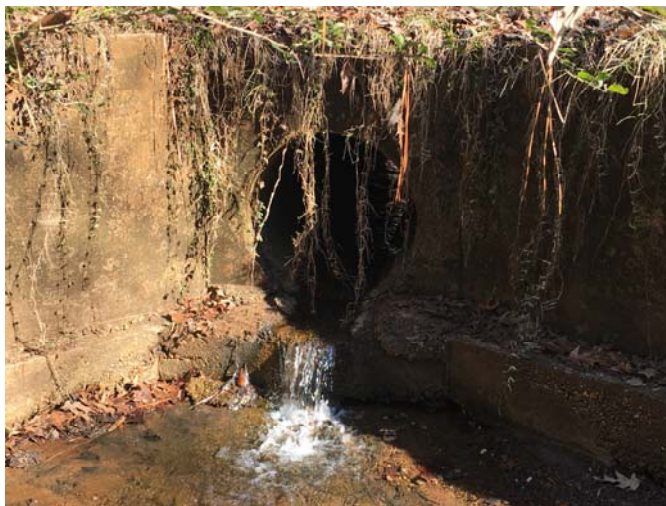
Photo 12 : Outlet of culvert, showing headwall encasing the culvert
