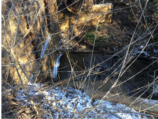
Photo 8: Upstream (east) side of road structure. Showing 48" dia CMP pipe.
