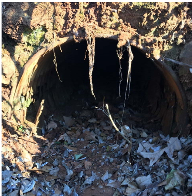
Photo 2: South end of Park St. culvert. Culvert is dry.
