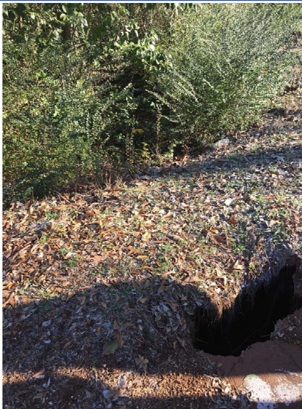
Photo: 3 North side of Park St. showing the culvert.
