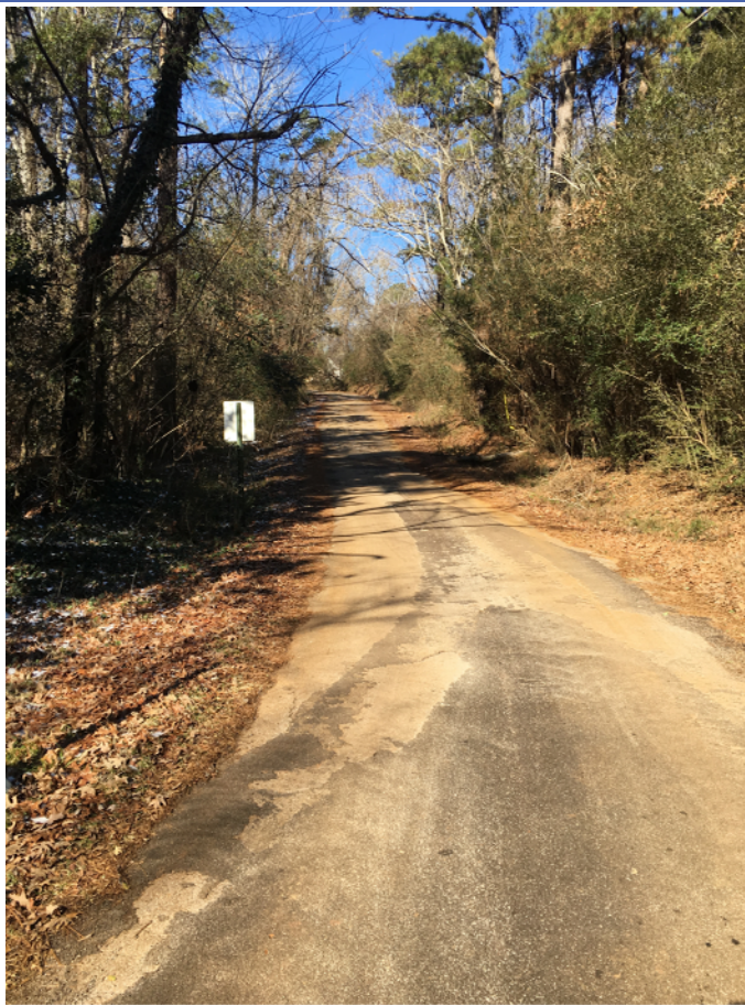
Photo 15: Bierhalter St looking west from the culvert
