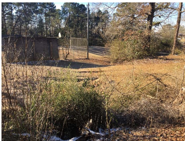
Photo 4: Park St. looking south (downhill) from damage site
